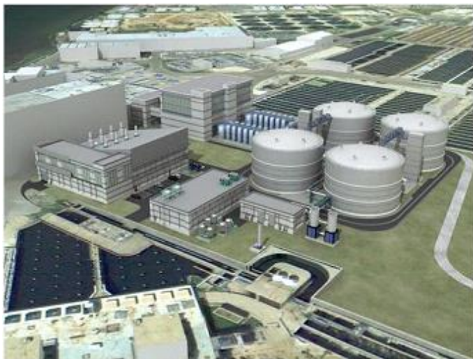
Figure 14: Cambi thermal hydrolysis and gas turbine CHP system at the Blue Plains facility
